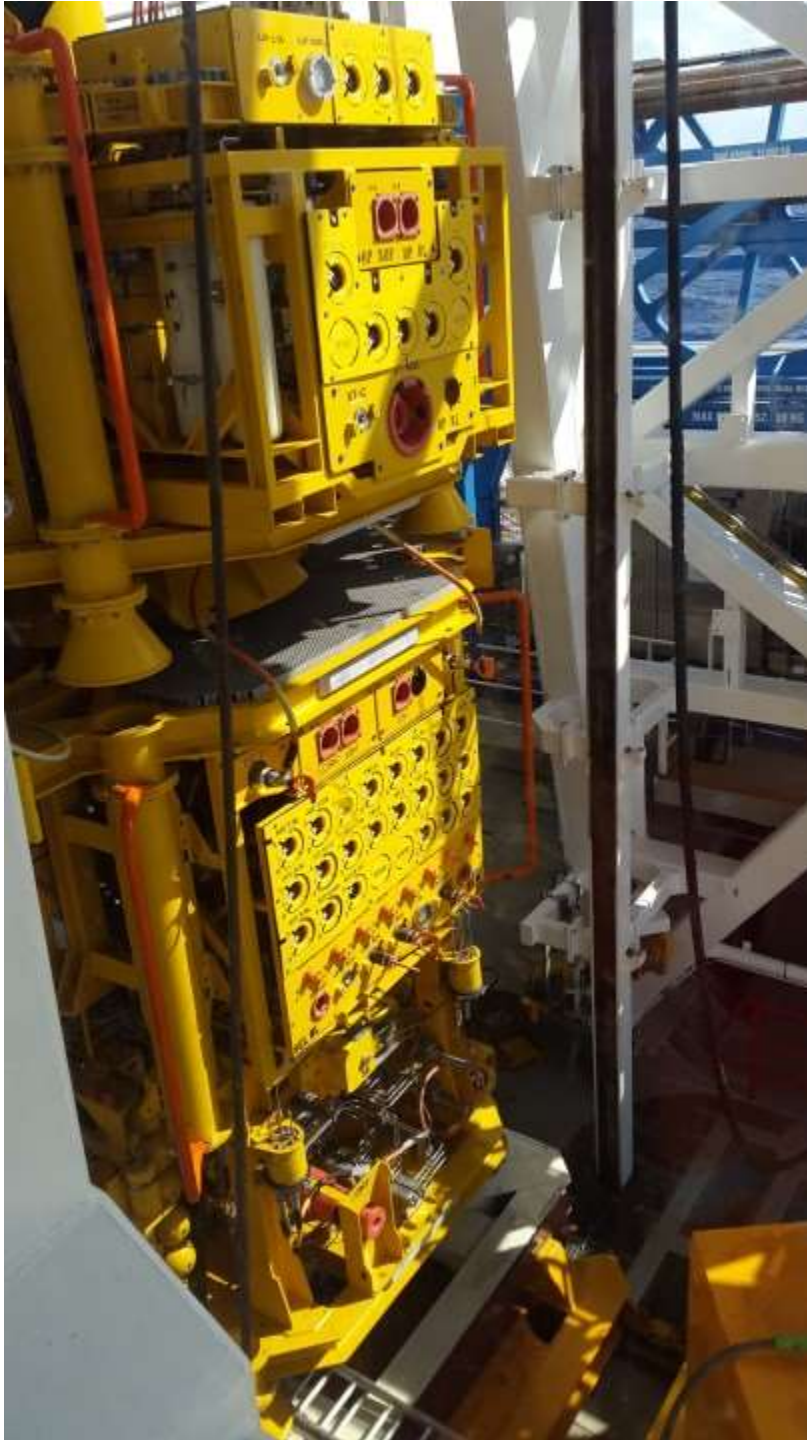
TFMC RLWI Stack 4 in the moonpool Island Performer 2015
