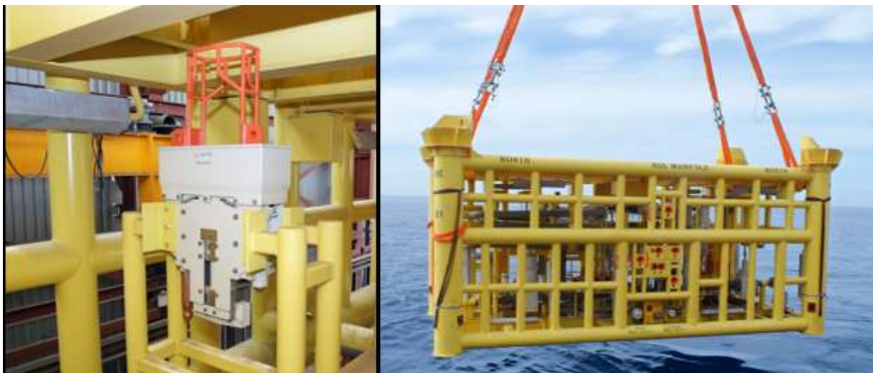
Figure 1: (Left) Preinstalled 2 inch female connector on a manifold, in the mated position; (Right) The manifold being deployed subsea.
